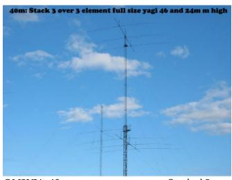
OM2VL's 40-meter antenna system. Stacked 3-element Yagis at 24m (80') and 46m. (150')
