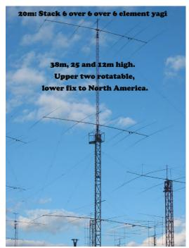
Laci's 20-meter system. Three stacked 6-element Yagis at 12m (40'), 25m (80'), and 38m. (125')
